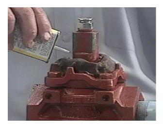
If the sealant is not being injected into the valve, use the valve flush purge compound to break up obstructions.
